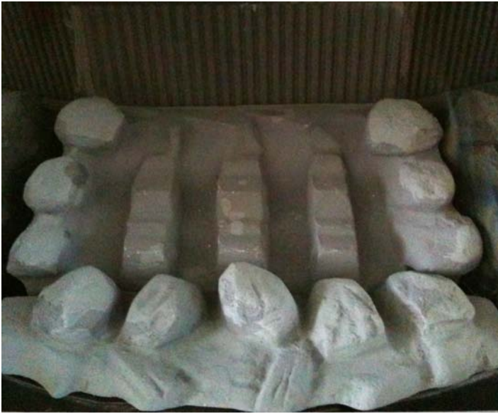
FRONT FIBRE SITS IN WELL OF BURNER AS ABOVE
